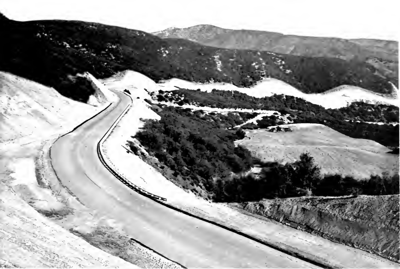
View of section of completed highway between Bradley and King City on U. S. 101 via Jolon, original route of El Camino Real.
